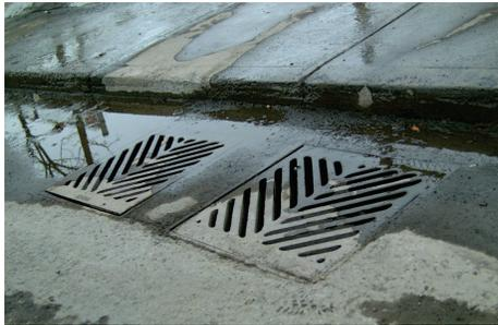
Storm drains (also referred to as storm sewers) are used to control stormwater runoff only. Stormwater runoff is water from the rain which flows from streets, lawns and rooftops over the ground or pavement without soaking into the ground. The storm drain system includes residential swale areas, roadside ditches, gutters, inlets, catch basins, and underground pipes that collect stormwater and carry it away from our streets, parking
